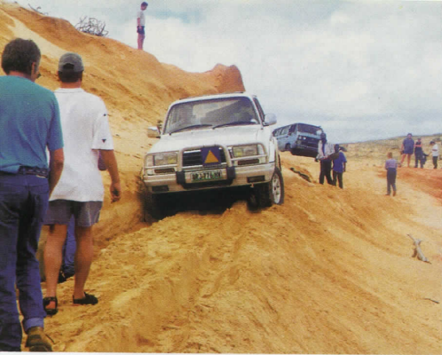
Left: Making a new road in Mozambique after the floods.
